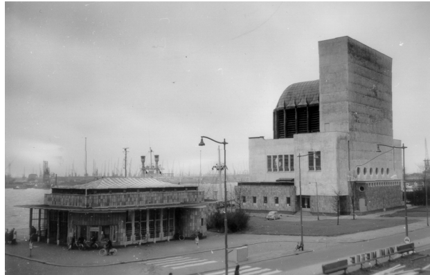
Rotterdam (Netherlands): Vent shaft building of the Maas tunnel 1965 (Source: testimon photo collection)
