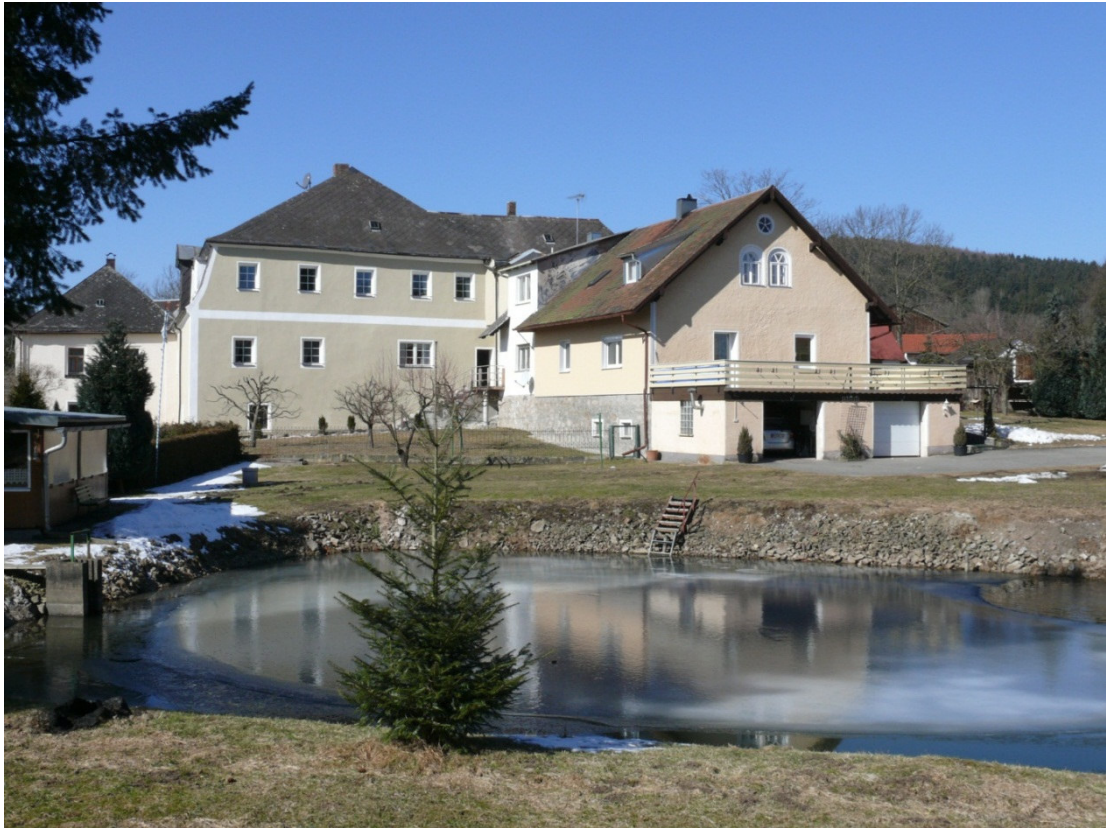
Figure 4: The former Frankenreuth manor house in 2011
