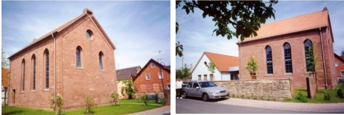
The restored former synagogue in Wiesenfeld, 1998 (photo: Ludwig Bauer)
