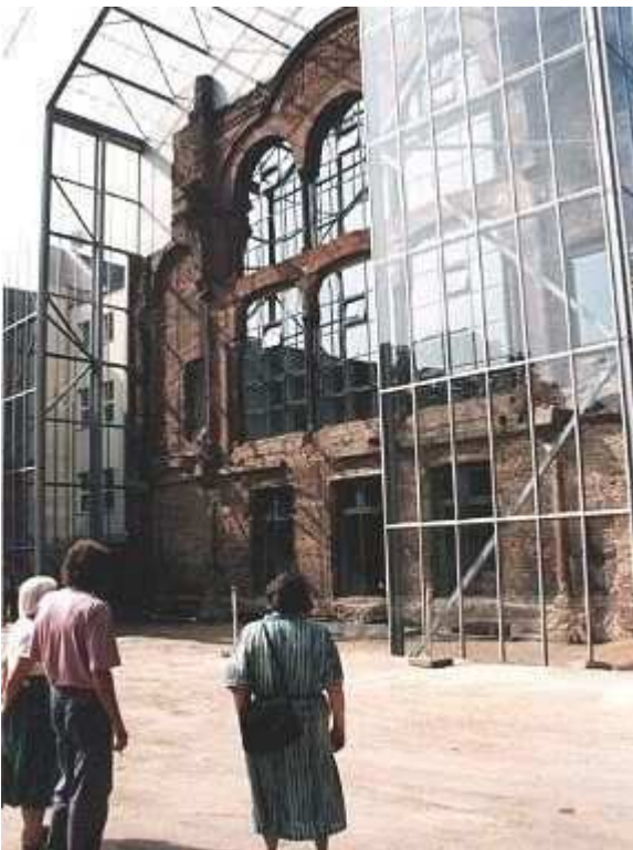
The back of the building. Nothing remained of the actual Synagogue, 1994
