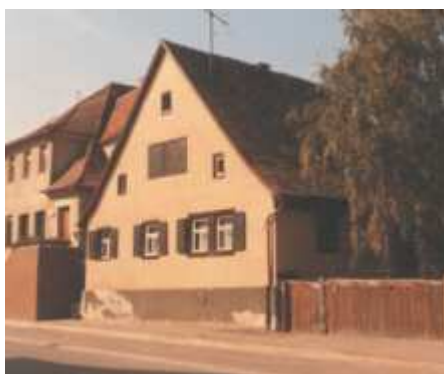
Hauptstrasse 27 (formerly house No 2), photograph of 1988
