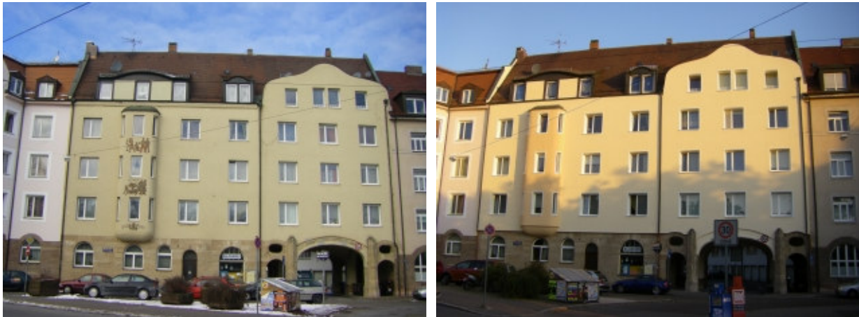
The façade at Platz der Opfer des Faschismus before (left) and after (right) its ‘cleansing’ (Photos: Susanne Rieger)
