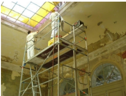
Restoration of the Leichenhalle (photo: Willie Glaser)
